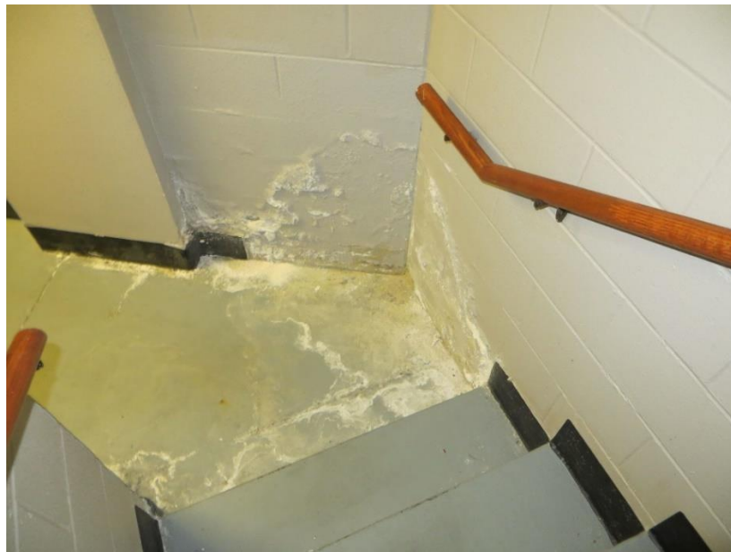
FIG. 18 EAST LOCKER ROOM STAIRS
