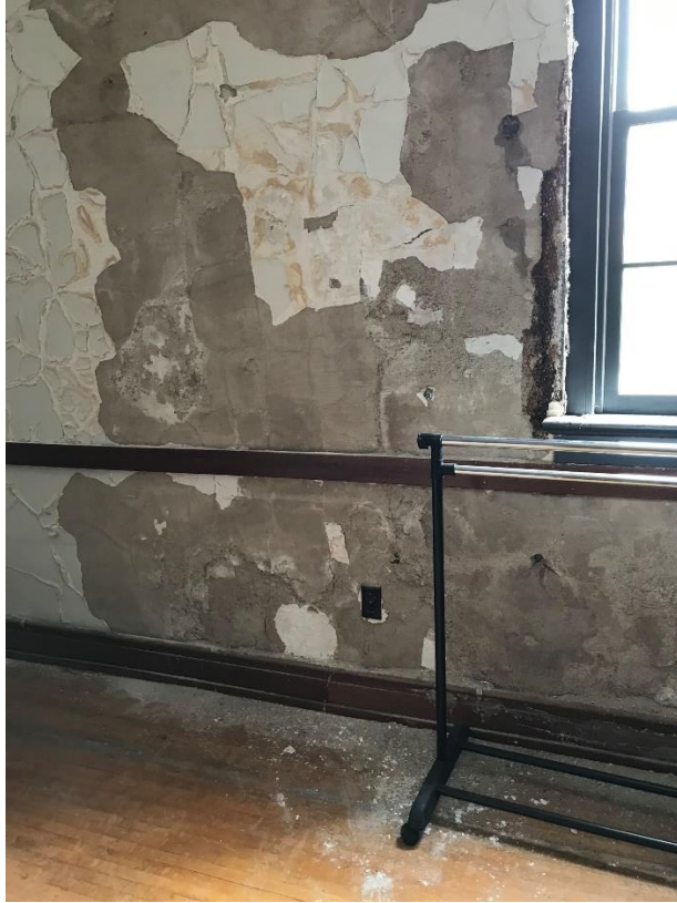
FIG. 14 PLASTER CRACKS ON SECOND FLOOR
