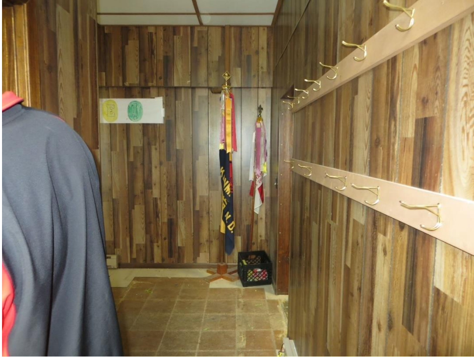
FIG. 13 EXISTING VCT FLOORING ON SECOND FLOOR
