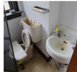
Figure 1- 2nd Floor Fixtures
