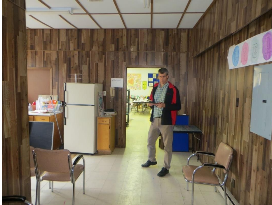
FIG. 15 WOOD PANELING WALLS ON SECOND FLOOR
