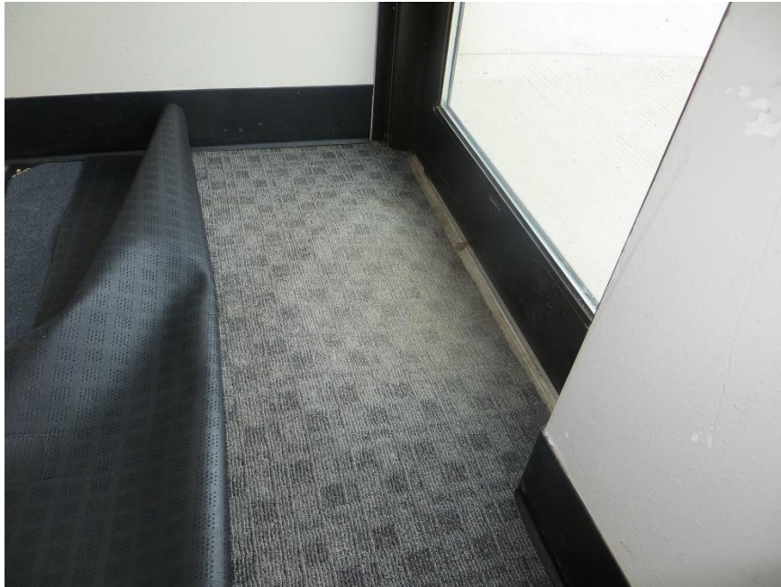
FIG. 9 CONCRETE FLOOR BUMP AT SOUTHEAST ENTRANCE
