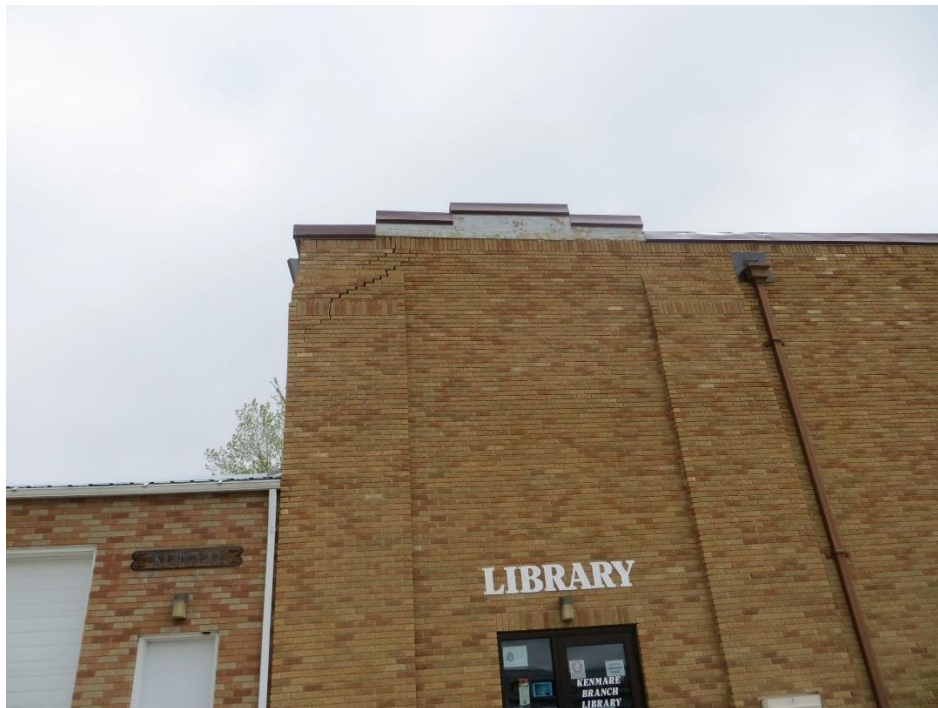
FIG. 4 NORTHWEST CORNER OF BUILDING
