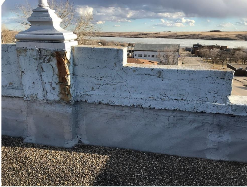
FIG. 7 BACK OF EXISTING STONE CAP
