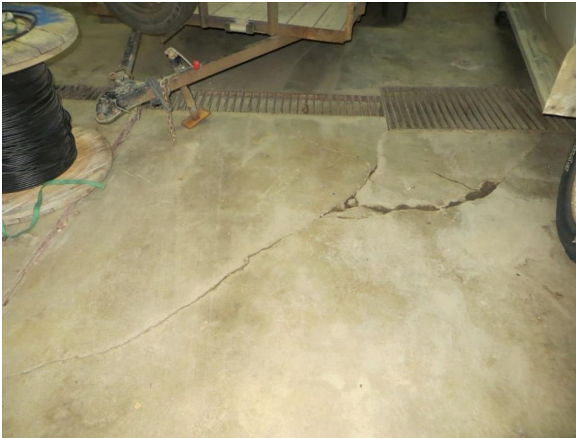
FIG. 11 GARAGE FLOOR CRACKS
