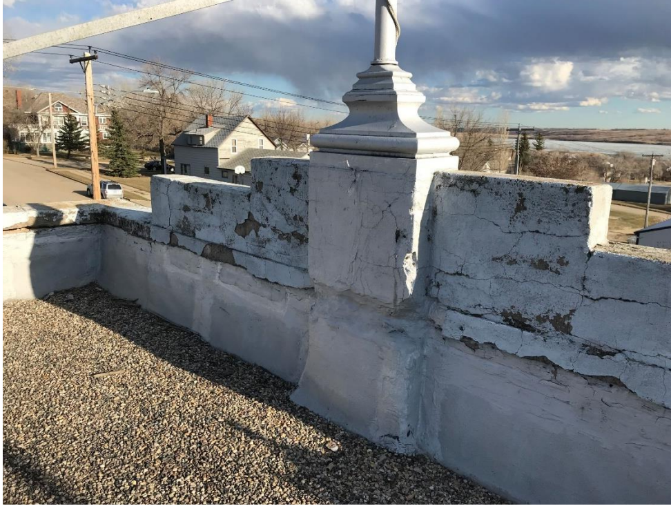
FIG. 6 BACK OF EXISTING STONE FLAG CAP
