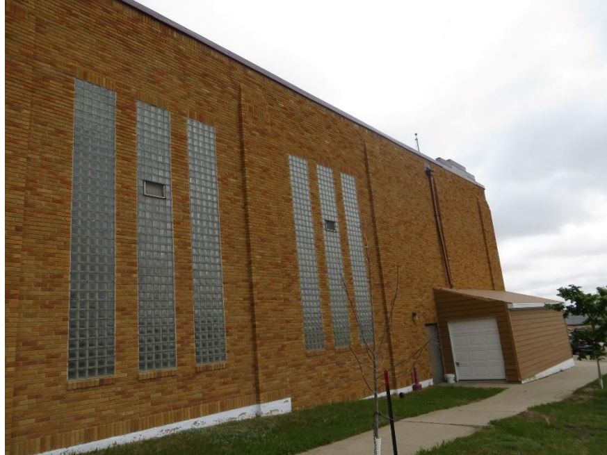
FIG. 17 EXISTING GLASS BLOCK WINDOWS AT WEST SIDE OF GYMNASIUM
